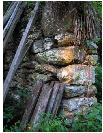
Mill Rock Wall
